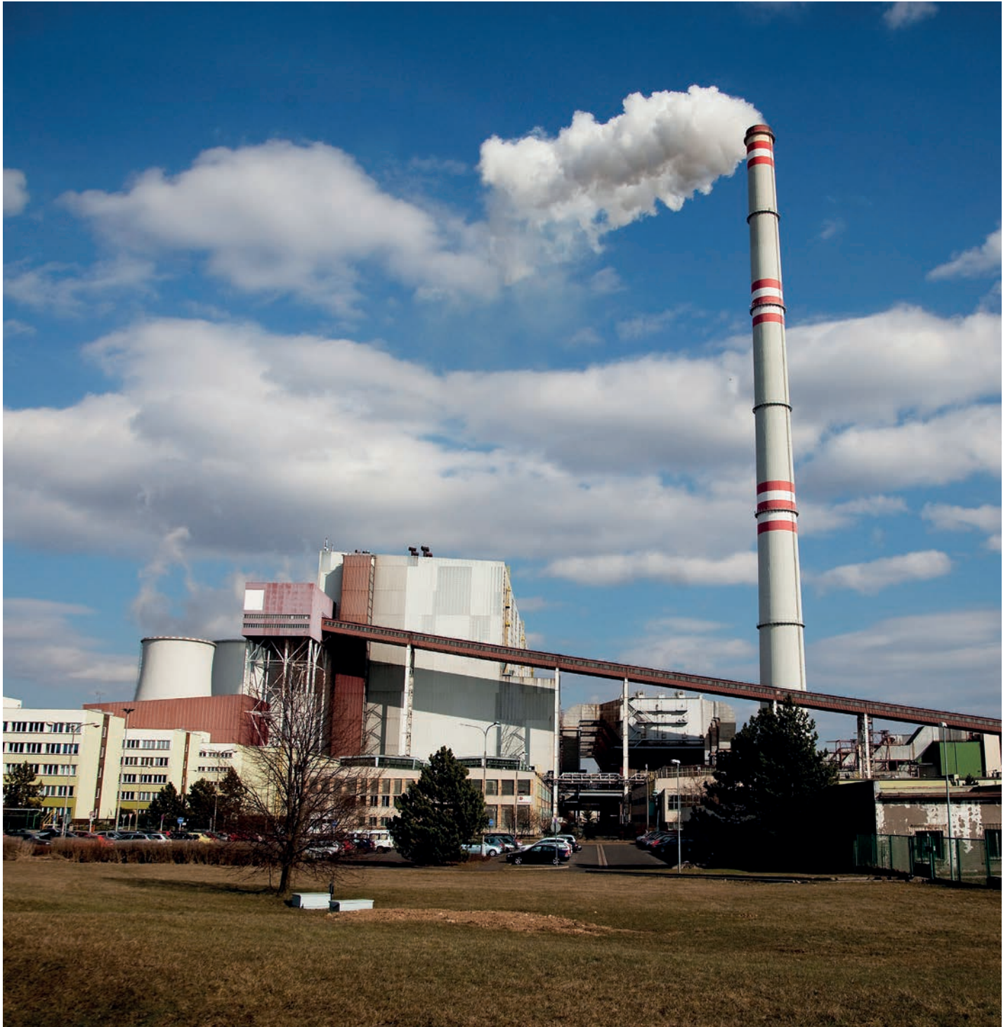
Prunéřov power station, Czech Republic. There is very little room for further technology-driven cost reductions for conventional power stations. Hence, future cost trends for fossil-fired power will be determined by fuel costs, carbon prices, and running hours (capacity factors).
